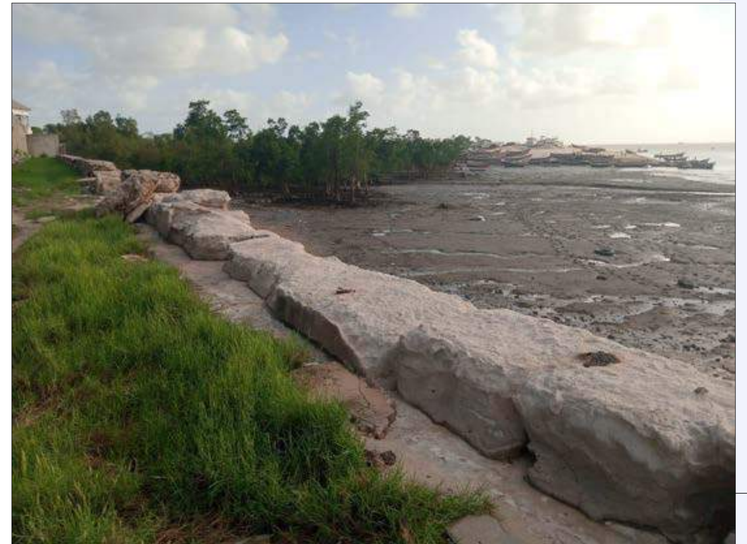
View of/from downtown seawall, looking south at Praia Nova
